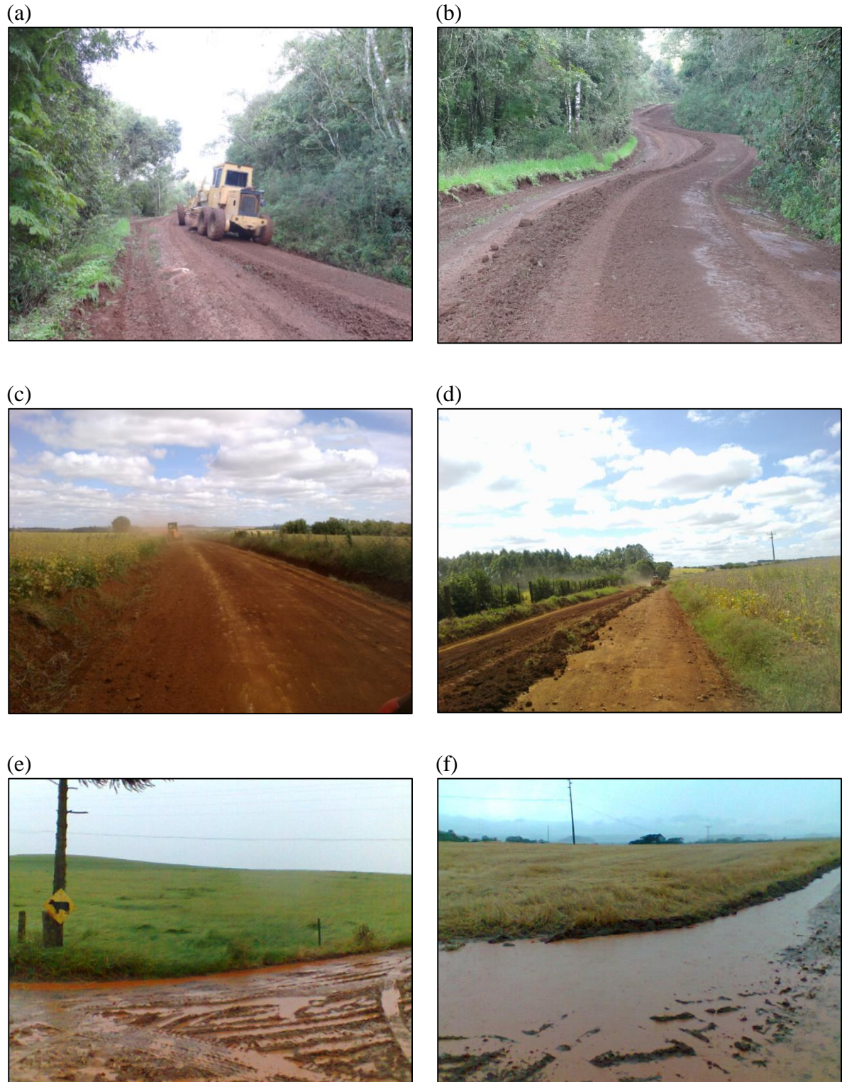
Figure 66 – Rectification of unpaved roads at Guaporé (a, b) and Conceição (c, d) catchments, and damages on unpaved roads structure induced by heavy agricultural machinery traffic under high humidity conditions (e, f).
