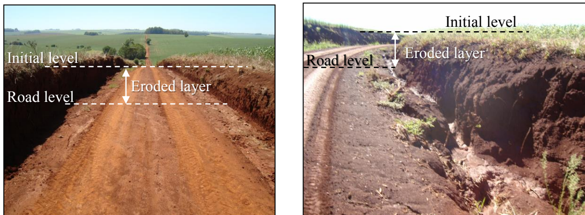
Figure 71 – Comparison of current roads level and the initial level of surrounding cropfields in Conceição catchment.
