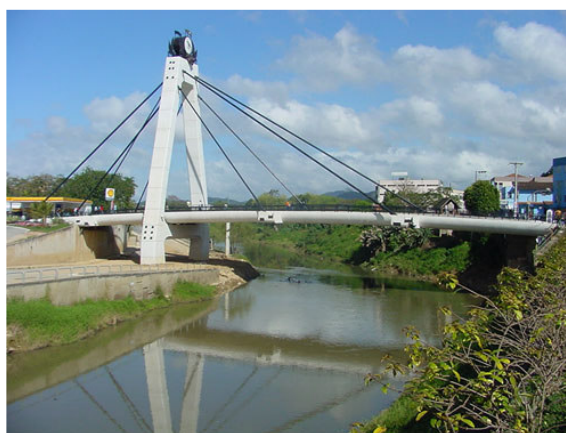
Figura 5.5 – Ponte Irineu Bornhausen, Brusque/SC
