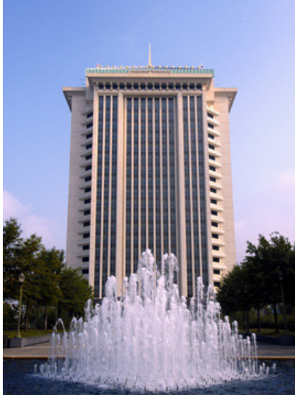
Figura 5.7 – RSA Tower Montgomery, Alabama/EUA Fonte: www.castonecorp.com/portfolio/rsa.html
