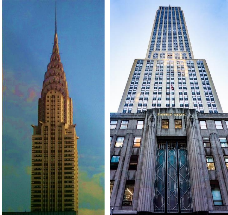
Figura 11 - (a) Chrysler Building ; (b) Empire State Building .
