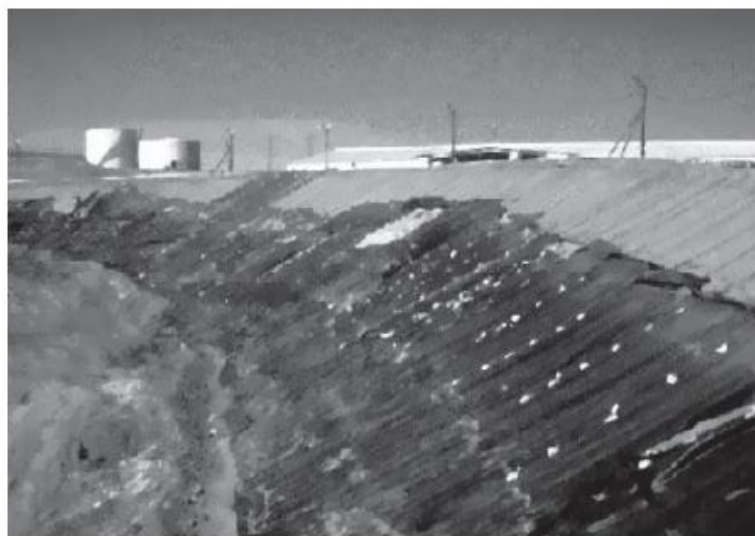
Figura 3 – Ruptura do aterro de Kettleman Hills.
