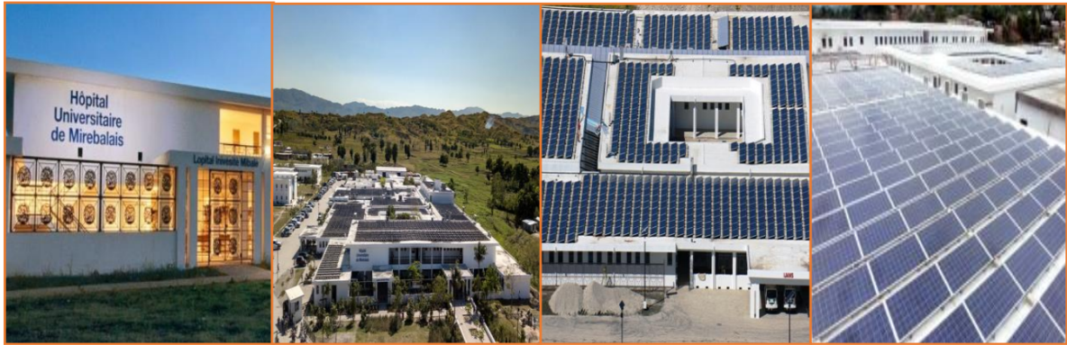
Figure 3.12 – University Hospital of Mirebalais, Area Centre of Haiti
