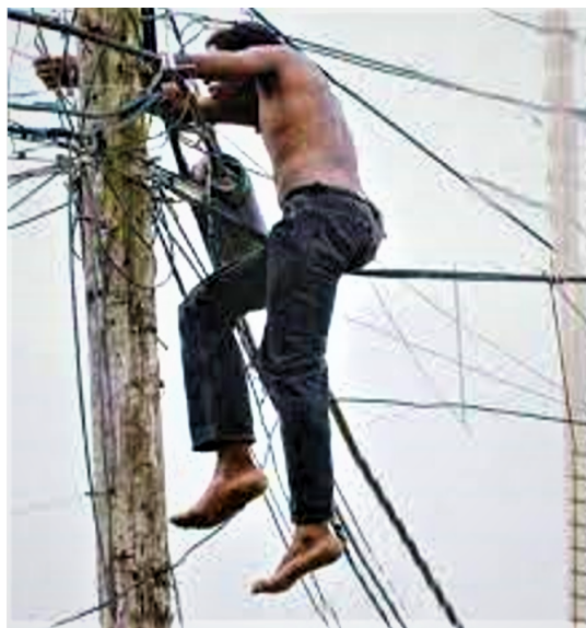
Figure 2.24 – Clandestine connection on the EDH network
