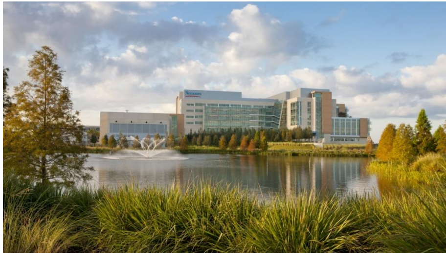
Figura 5 - Vista geral - Nemours Children's Hospital
