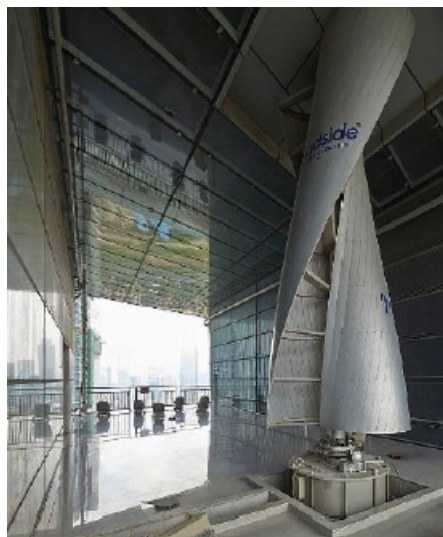
Figure 2.17 – Wind turbine inside air conducts.
