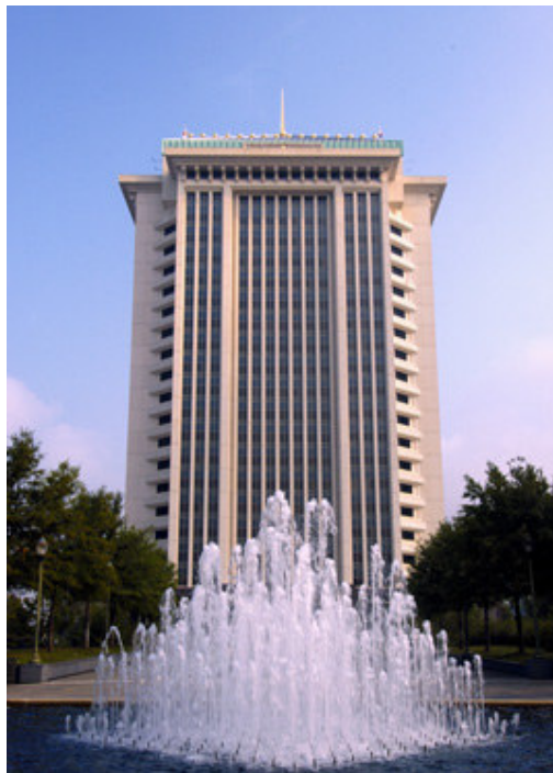
Figura 3.1: RSA Tower Montgomery, Alabama, EUA - Fonte: http://www.castonecorp.com/portfolio.html
