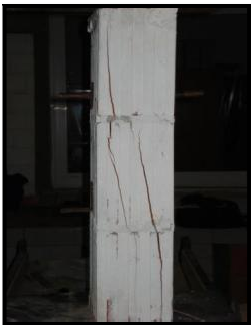
Figura E9: Prisma de 3 blocos T1BPV
