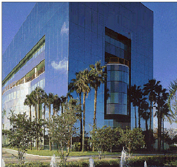
Figura 23 – Fachada “Structural Glazing”
